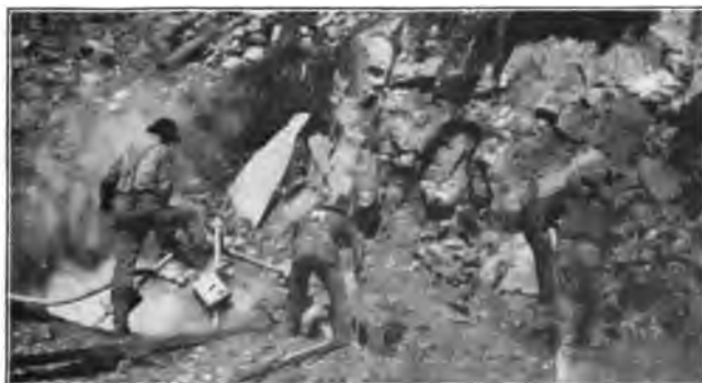
C. STARTING EXCAVATION FOR SHAFT AT SOUTH LAKE MINE, 1912.
